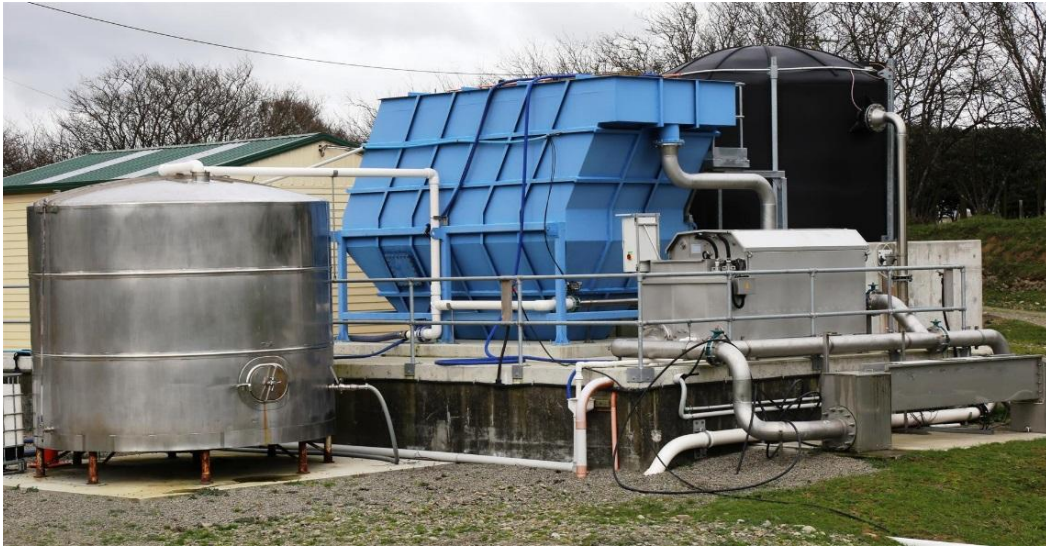
Figure 2- Lamella Filter, Coagulant Tank, uv Micro-filter and Sludge Tank
